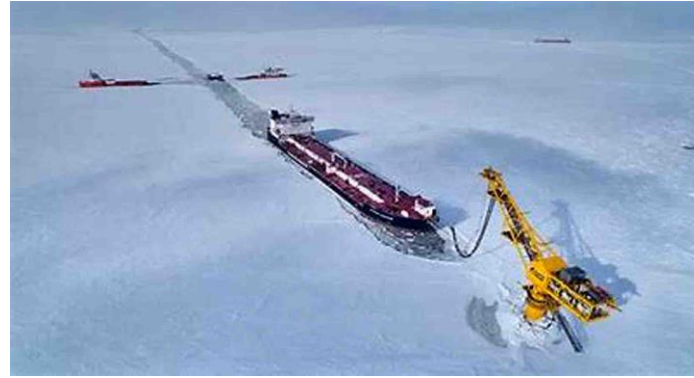
Oil Pipeline and Export Terminal
