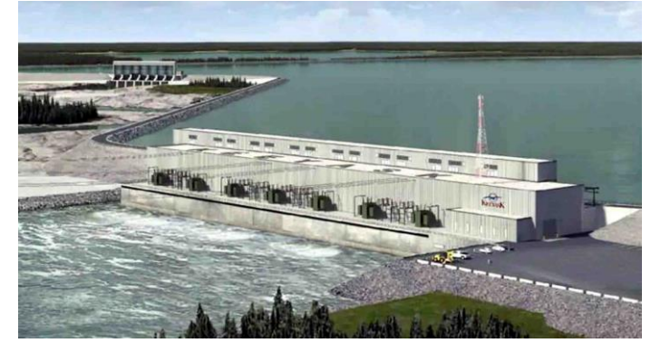
Hydro Electric Transmission
