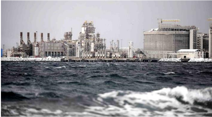
Natural Gas Pipeline and LNG Facility
